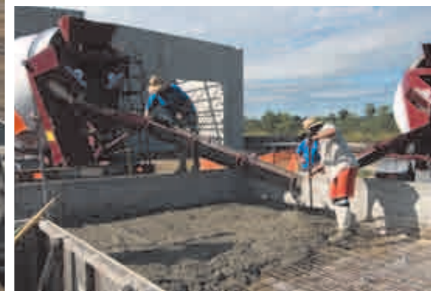
Left and top: Preparing the on-site precast bays with ONEMESH®, REBAR and accessories at Yatala Business Park development, Queensland Above: Pouring one of the 300 tilt-up panels required for the project.
