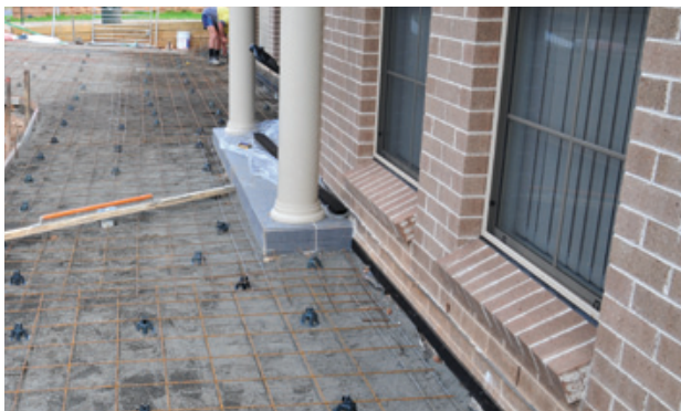
The compact 4 m x 2 m sheets can be used economically in projects for driveways and paths offering savings in material.
